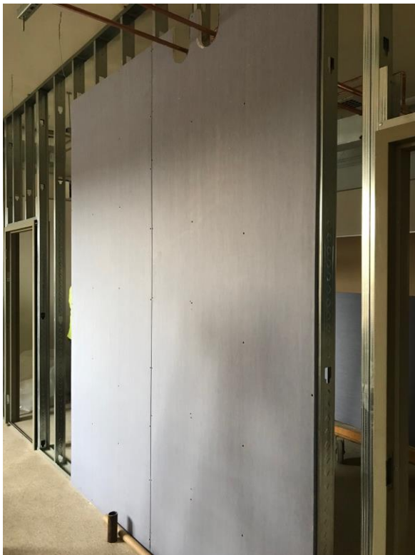
Sheetrock Installation
