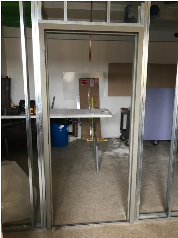
Installed Door Frame
